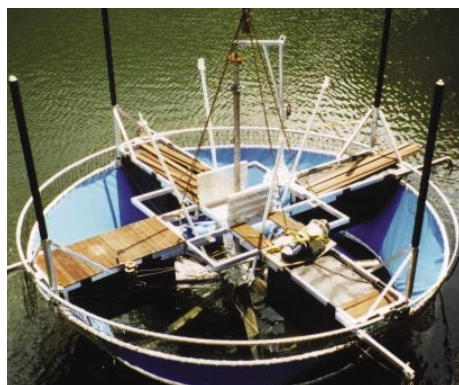
A reservoir mixer unit being installed. Once assembled, the unit floats with the impeller immersed and is tethered to the bottom of the reservoir
