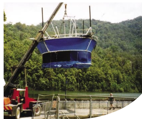
A reservoir mixer unit being installed. Once assembled, the unit floats with the impeller immersed and is tethered to the bottom of the reservoir
