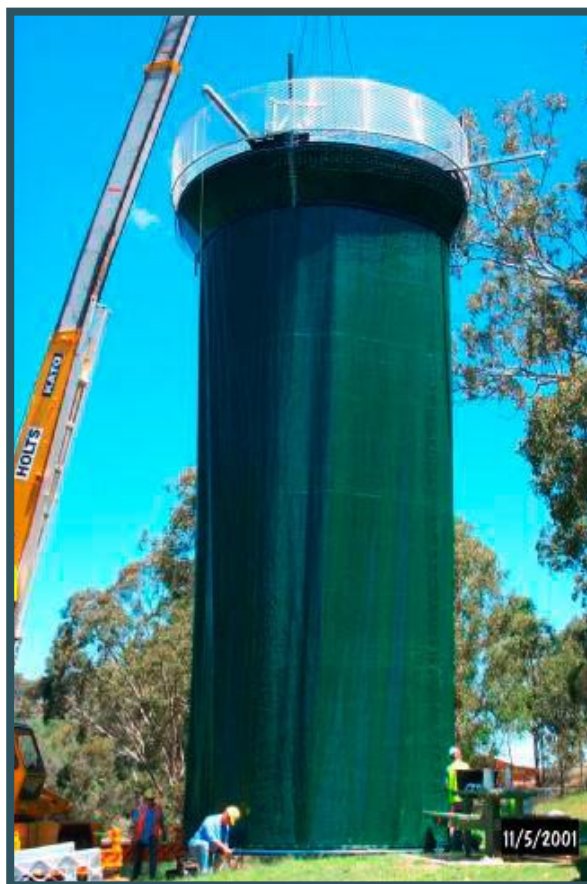
Figure 9. One of the WEARS SMDI-5s, to be coupled with another, being prepared for installation at Cooby Dam for the Toowoomba City Council.
